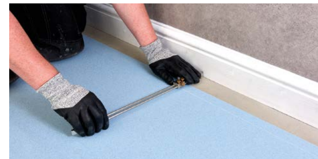
Figure 2 Scribing the wall profile
