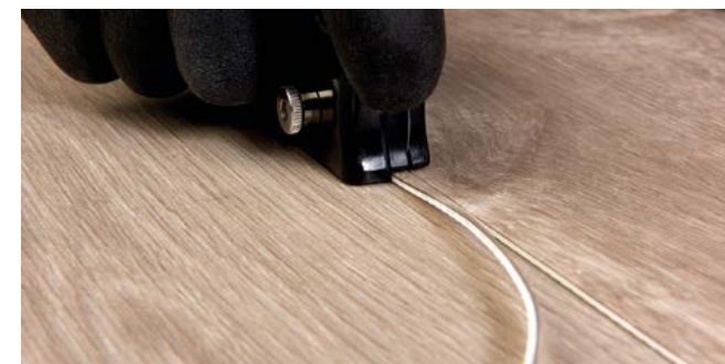
Figure 5 Cutting in the seams
