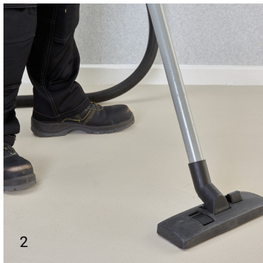
2 Sweep or vacuum the floor area, check the condition of the subfloor and make good as necessary. If the substrate is highly porous a suitable primer may be required.
